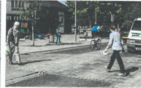
Example of setts being used to define a courtesy crossing
