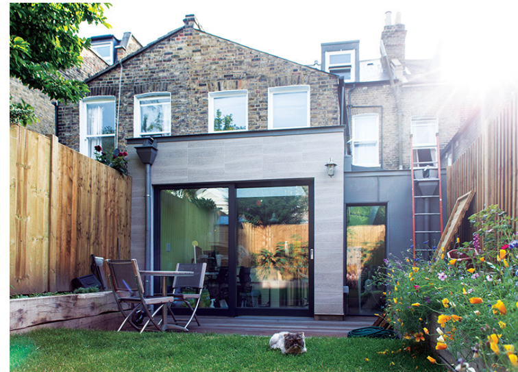
EnerPHit retrofit project with extension (Source: Passivhaus Plus)
