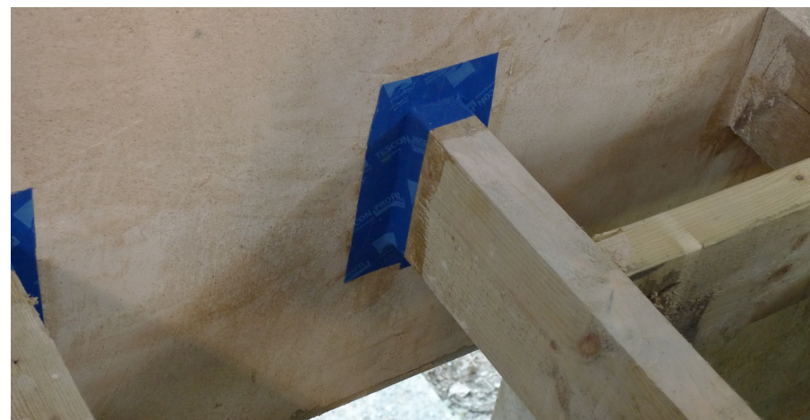
Applying airtightness tape to joist ends is a common measure required to achieve good airtightness in existing buildings. Large gaps may need filling with mortar first, and remember to apply a suitable primer. (Source: Ecomerchant)
