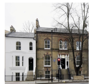
Akerman Road, London (Source: 15-40 Architecture)
